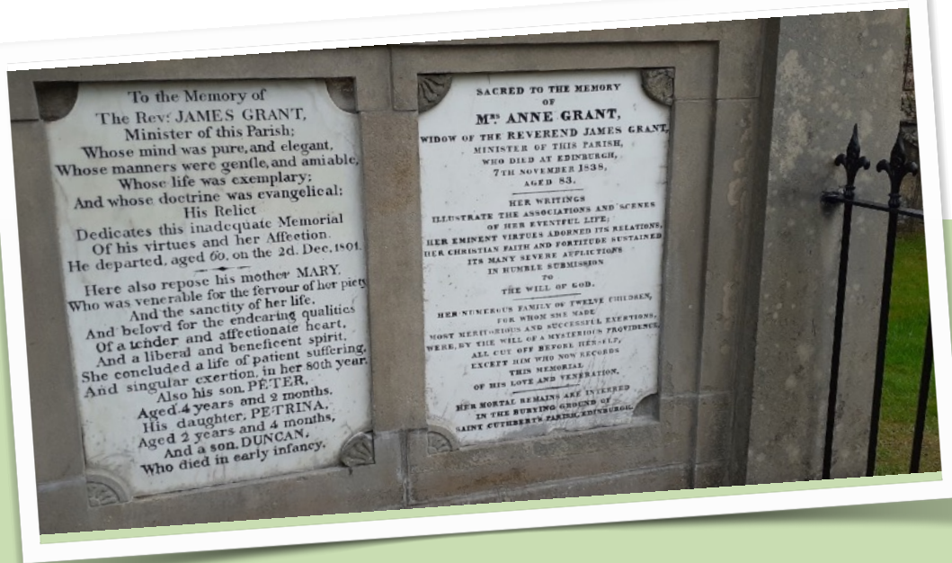
Repaired stone photo by Graham Grant
