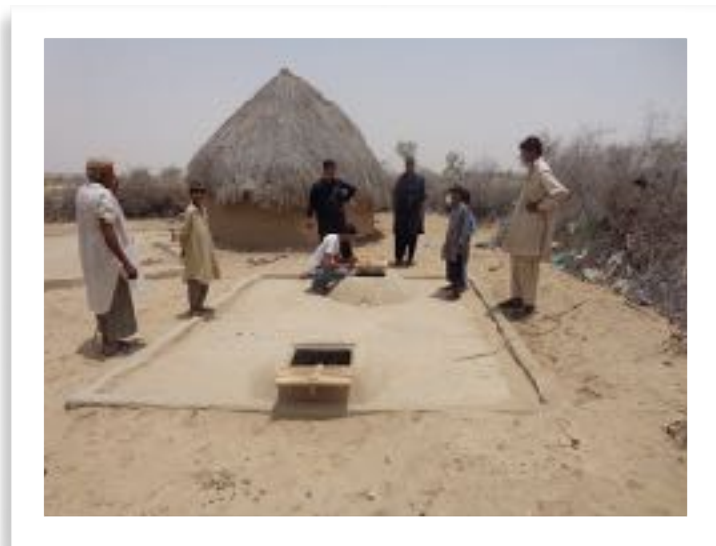
Underground storage tanks in the Thar Desert, Pakistan.
