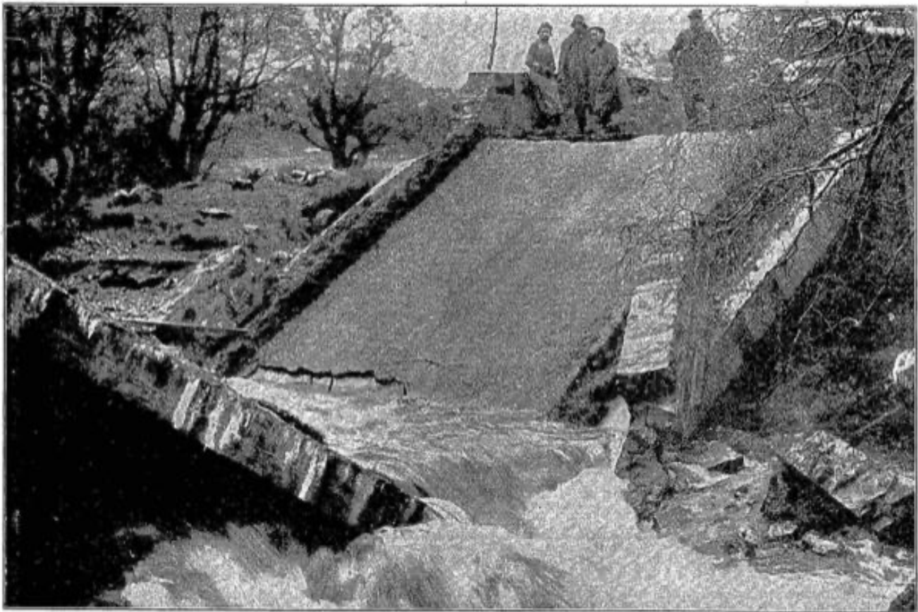
HIGHLAND BRIDGE DOWN. —Aberarder Bridge, Loch Laggan-side, on the Kingussie-Fort William road, which has collapsed owing to the subsidence of a centre column following a spate. All traffic was stopped at the week-end.
